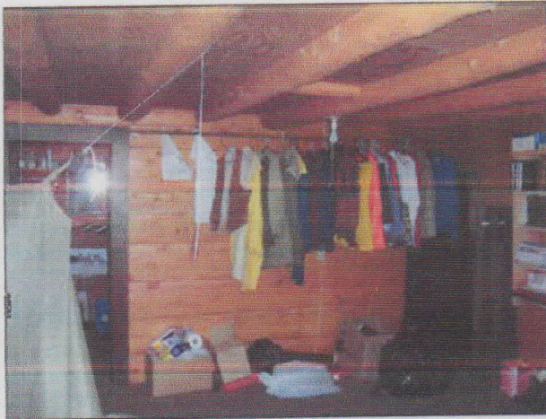
Interior of Building #6
