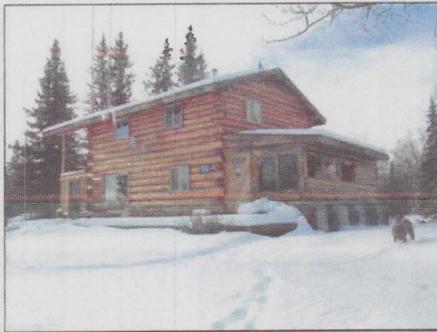
Looking SW from the bank at the front elevation of Building #12
