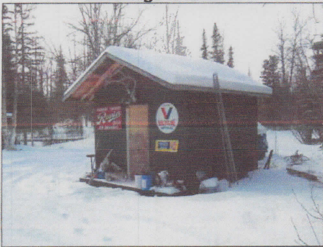
Building #13 - plywood shed
