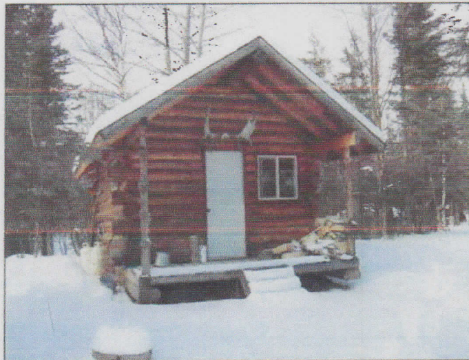
Building #18; an outhouse (#19 is not shown)
