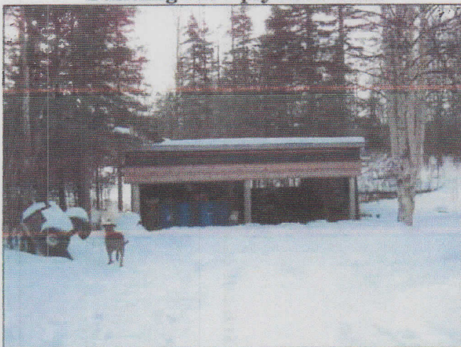
Building #16 - pole shed
