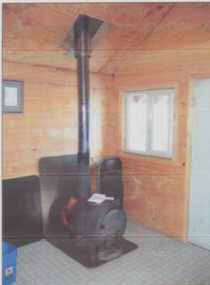
Interior of Building #18
