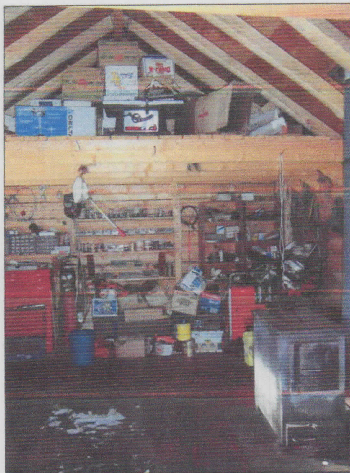
Interior of Building #3
